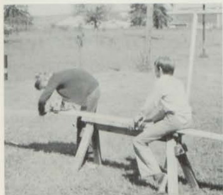
Building A Storage House
