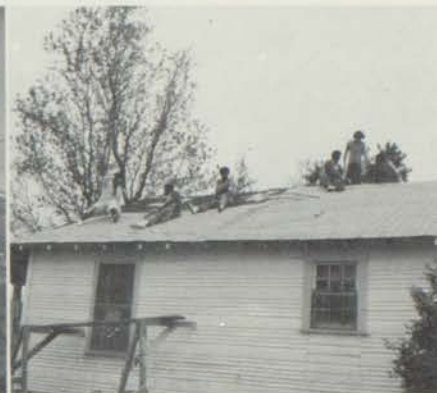
Repairing A Roof
