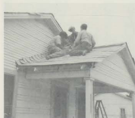
Shingling A Roof
