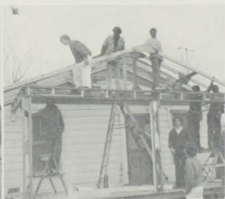
Replacing A Porch
