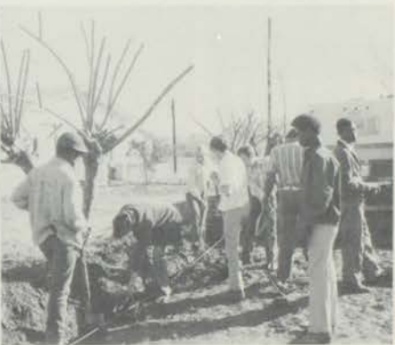
Grading A Driveway
