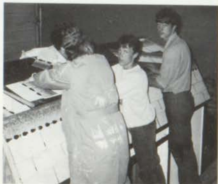
Anthony Starnes, Billy Allen, Steven Adcock roofing a storage bldg.
