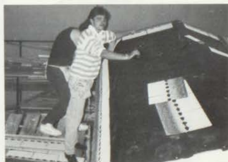
Callen Neff, Jamey McIntosh roofing a storage bldg.
