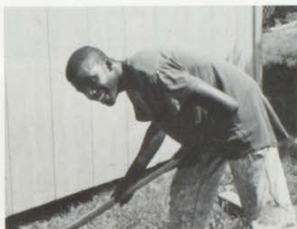
Rodney Talbert leveling a storage bldg.
