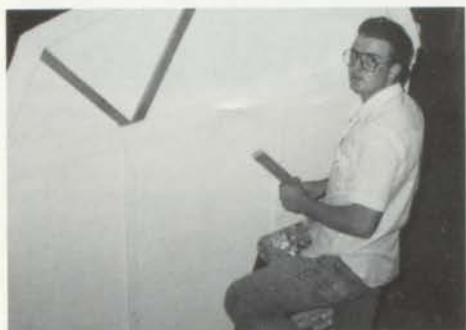
Danny Neff installing trim on the storage bldg.
