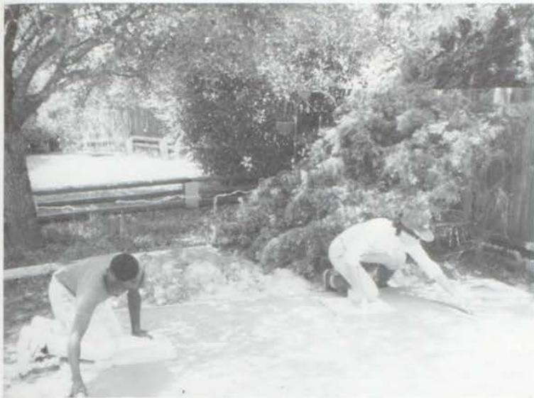
Quincy Mitchell and John Shaw finishing concrete
