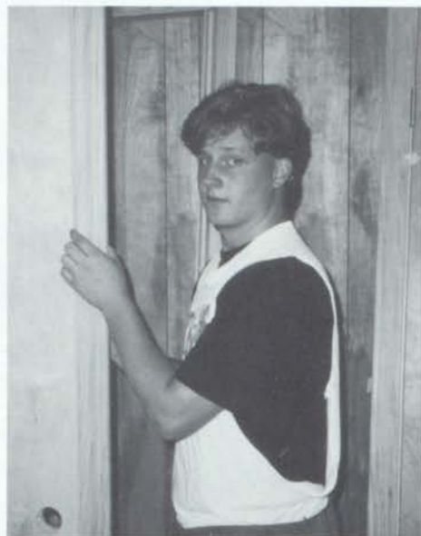
Jason Hopkins hanging a door unit.
