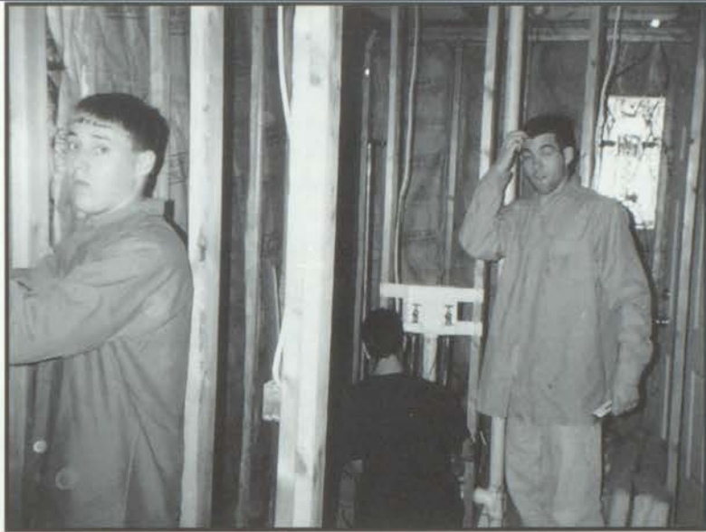
Reuben Spears and Derek May install electrical wiring in the house.
