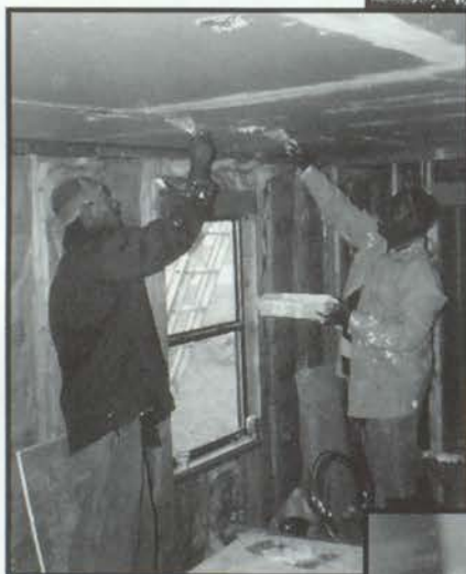
Jamie Traylor and Otis Richards trap and bed the sheetrock.
