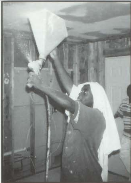
Ryan Wade blows the ceiling texture on the ceiling.
