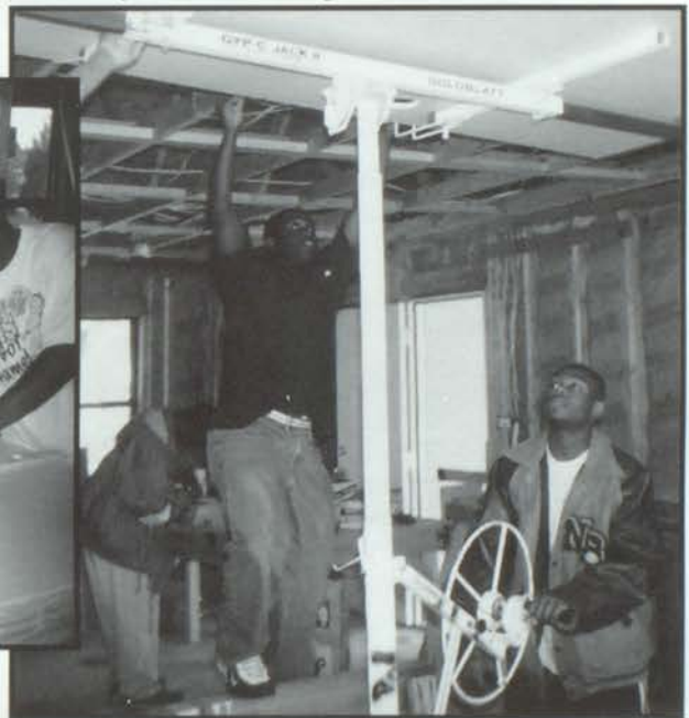
Horatio McChester helps Ryan Wade hang sheetrock.
