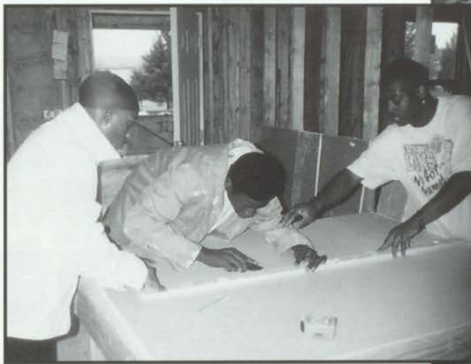
► Jason Cribbs, Marcus Stephens, and Shaundre Burns cut the sheetrock for the ceiling.
