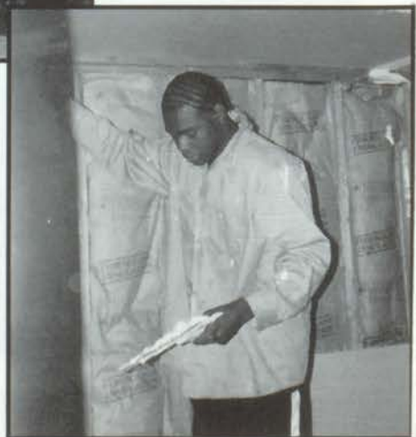
► Ronnie Walker finishes sheetrocking the house.
